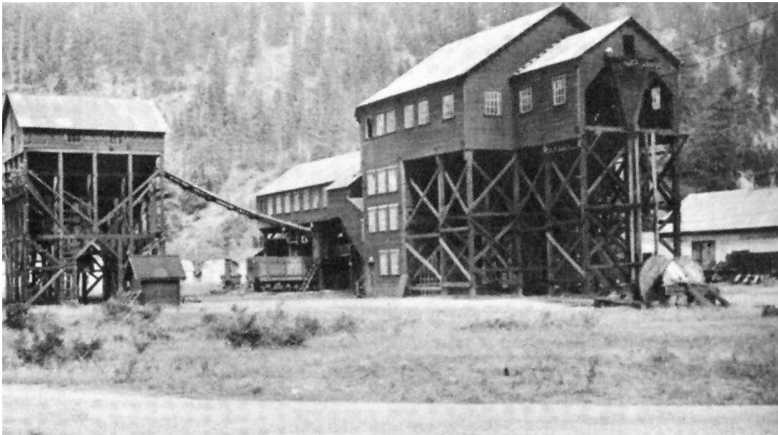
Coalmont Tipple – End of the run for the four-mile aerial tramway
