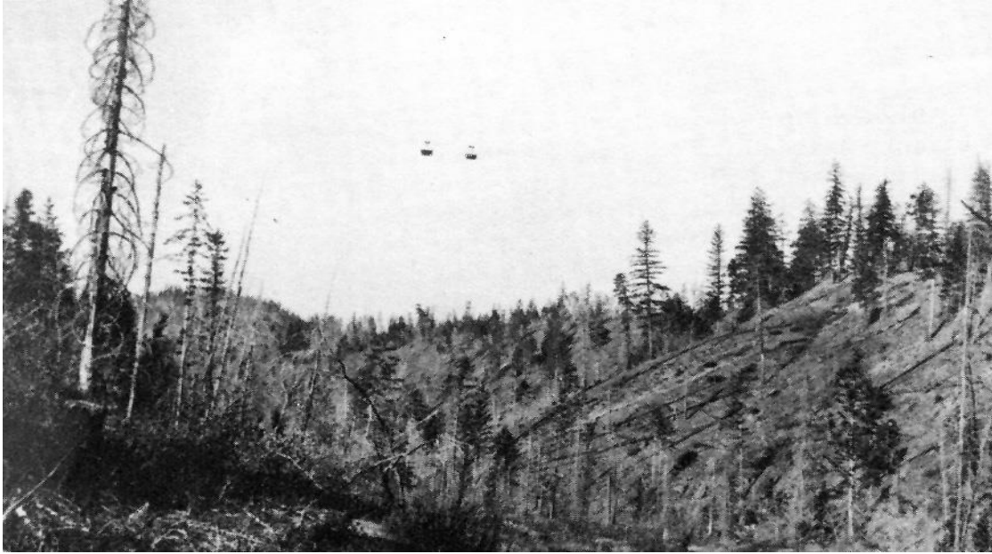
Tramline buckets over the Canyon prior to Anchor Hill
