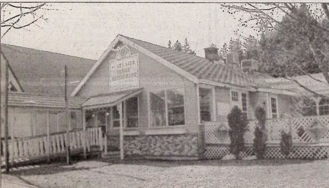
The historic mine rescue building on Vermilion Avenue has gone through many changes and has become an attractive restaurant featuring a summer patio under a shade tree.
