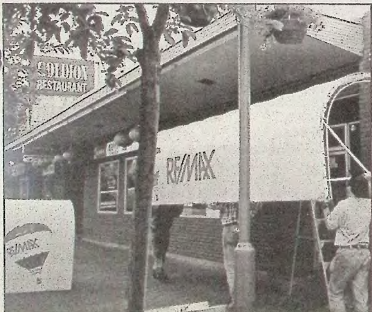
Re/Max has moved across the street. Above, workers take down the Re/Max canopy from the old location.
