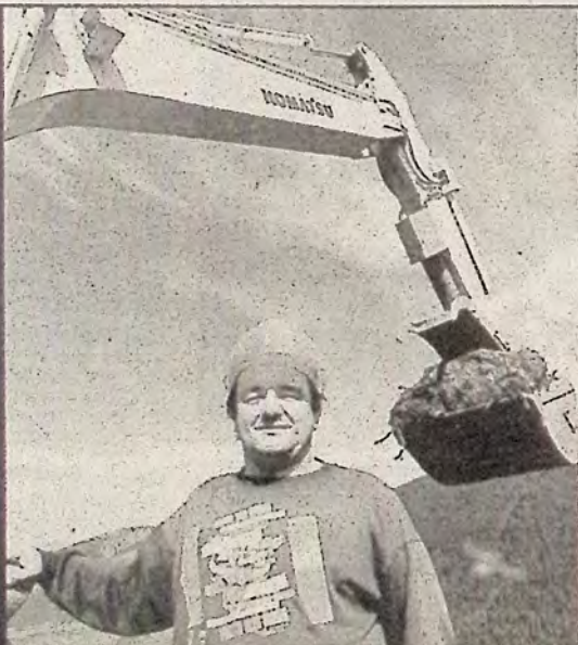
[Road deactivation in Horsefly area]
