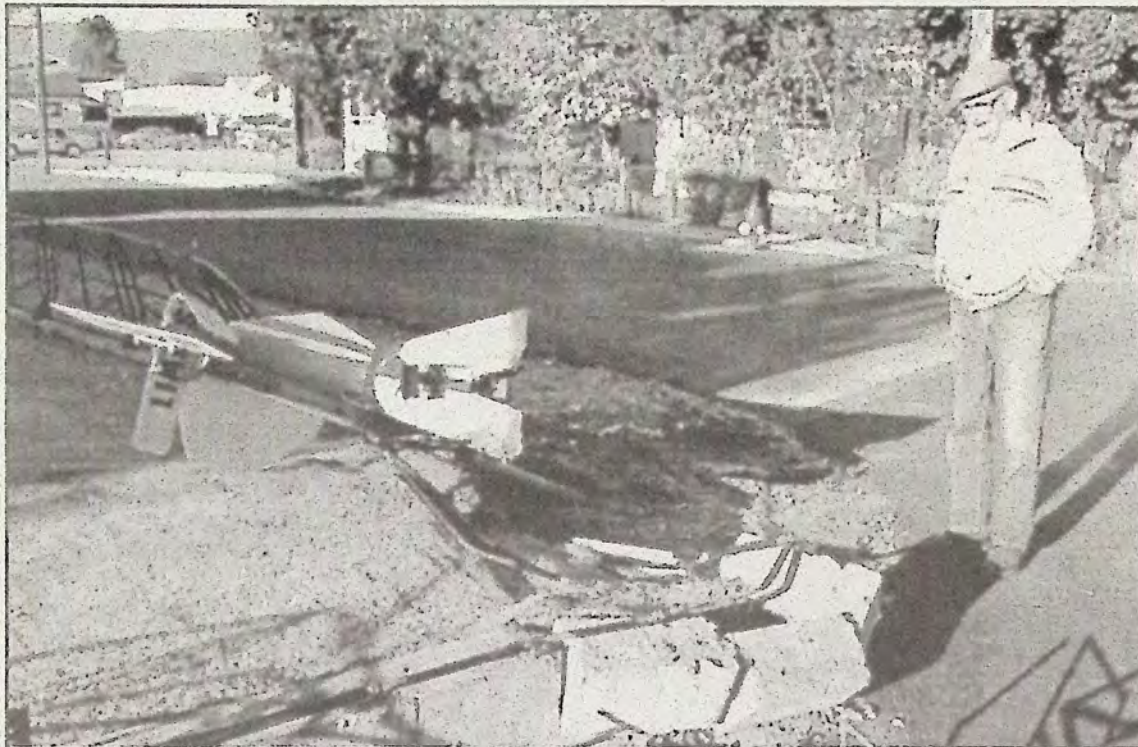
Bill Smith, who owns a home at the corner of Harold Avenue and Lime Street had his fence and retaining wall wrecked at 7:40 pm October 22. His wife, Ruby, rushed out to see a "huge light colored truck" going down the street. Smith was distressed to learn that repairing the damage will cost $2500 to $3000. Fortunately it is covered by insurance. The identity of the trucker is unknown.
