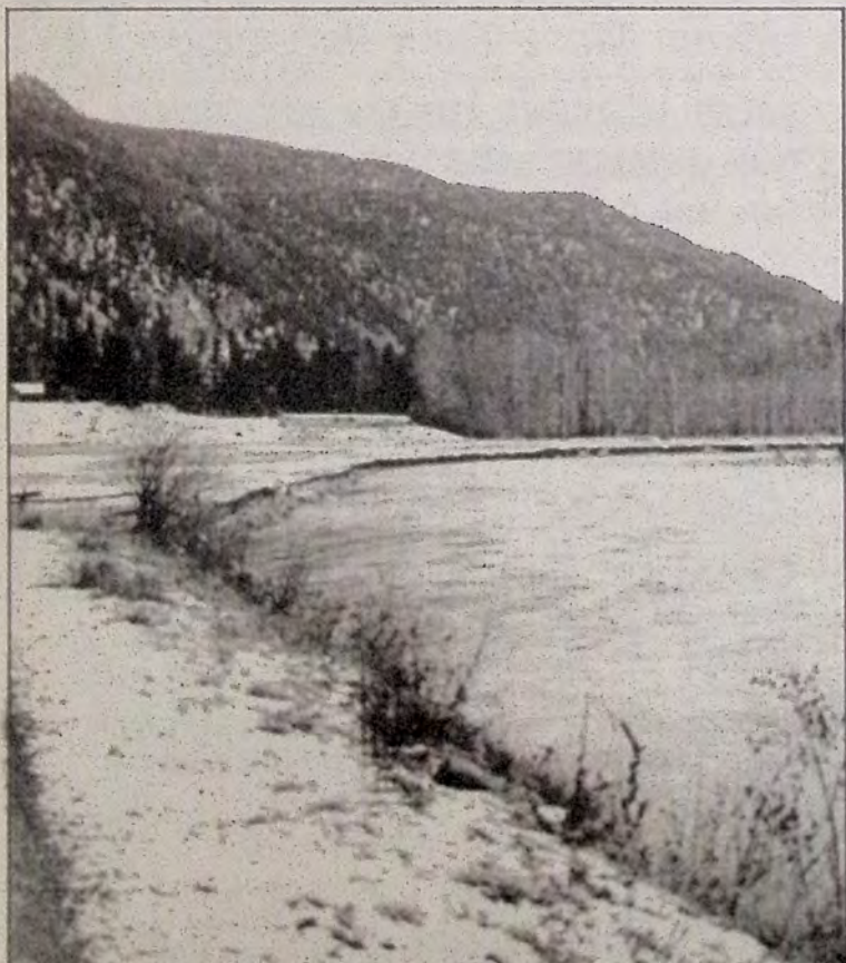
The dark line along the edge of the river shows where acres of good bottomland were swept away on this Indian Reserve land. Dikes are a provincial responsibility. Reserve lands are considered federal. There were no dikes to protect the Indian Reserve land.
