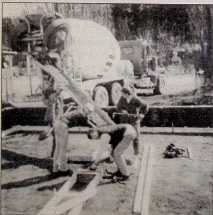
They're at it again in Tulameen - construction of new homes is underway. Three more housing starts are scheduled for this spring in Tulameen.
