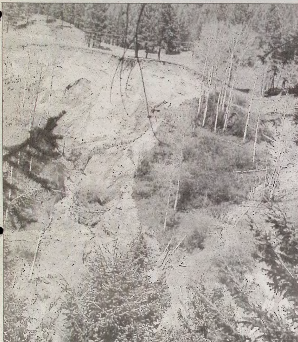
The collapsing hillside at the edge of Doug and Edith Currie's pasture shows the flow of mud down to Asp (China) Creek. Trees and bushes have fallen into the mud flow down the 100 metre slope.
