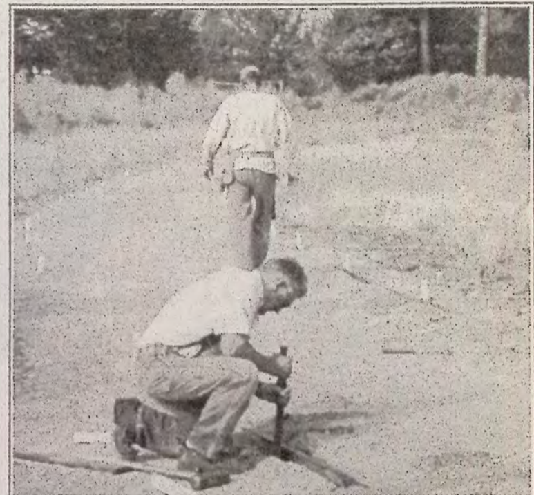
Cedar edging is pushed into place along the pathway.
