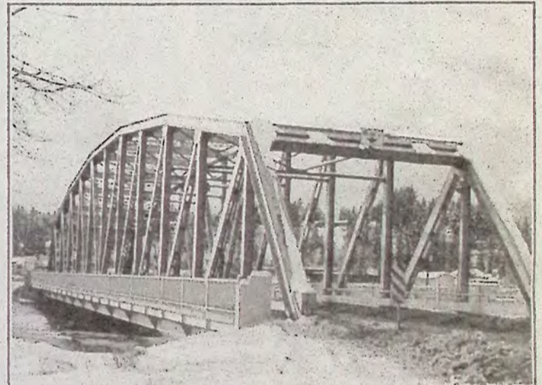
The blue bridge across the Similkameen River on Highway 3 is slated for replacement. Vermilion Trails Society has been asked if they would like parts of the bridge. Society members wonder what they could do with the bridge and which parts would be usable. They are considering the handrails and some girders they feel might be useful.
