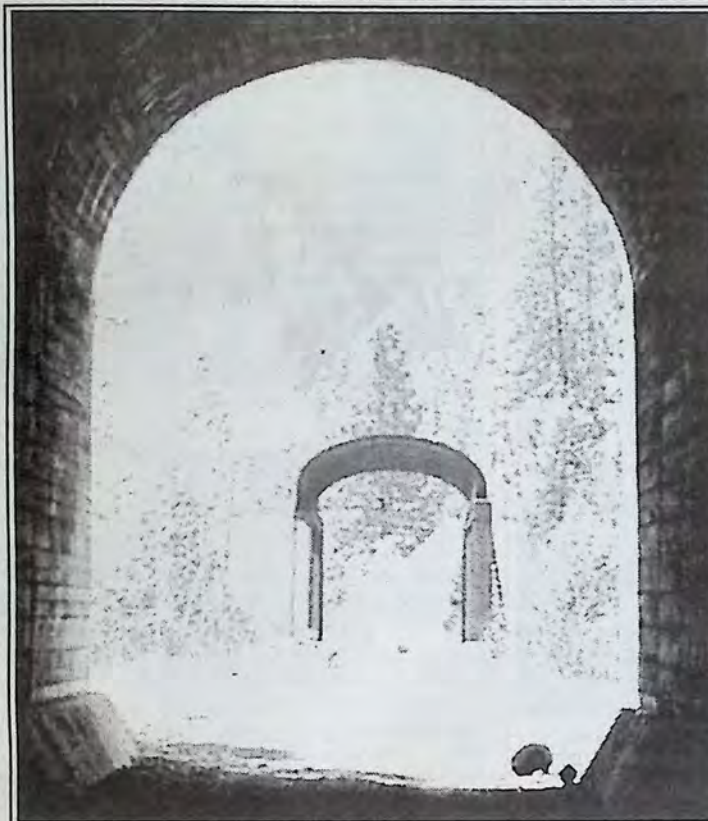
The water carrier will come across the bridge over the Tulameen River, through this tunnel, and follow the trail to downtown Princeton.
