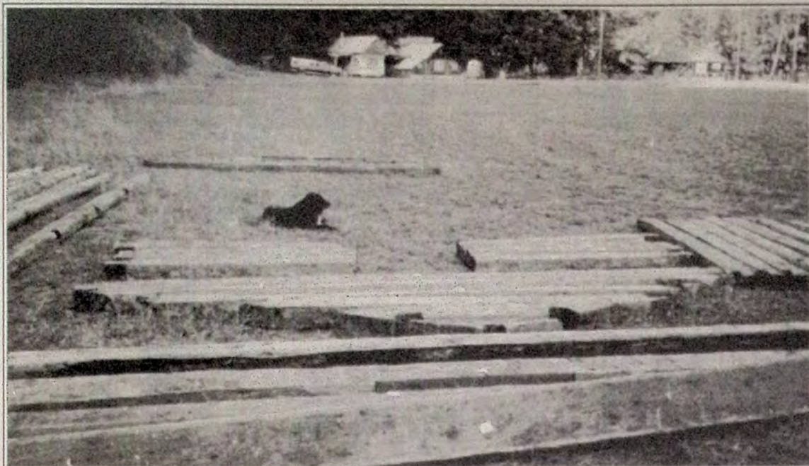
The old schoolhouse in Tulameen is on the move. Above, the logs are being dismantled and tagged, one by one, for re-assembling at the new site where it will be a museum. The dog took a protective, if puzzled, attitude toward the venture, and watched every move. Photo by Anne Passey.
