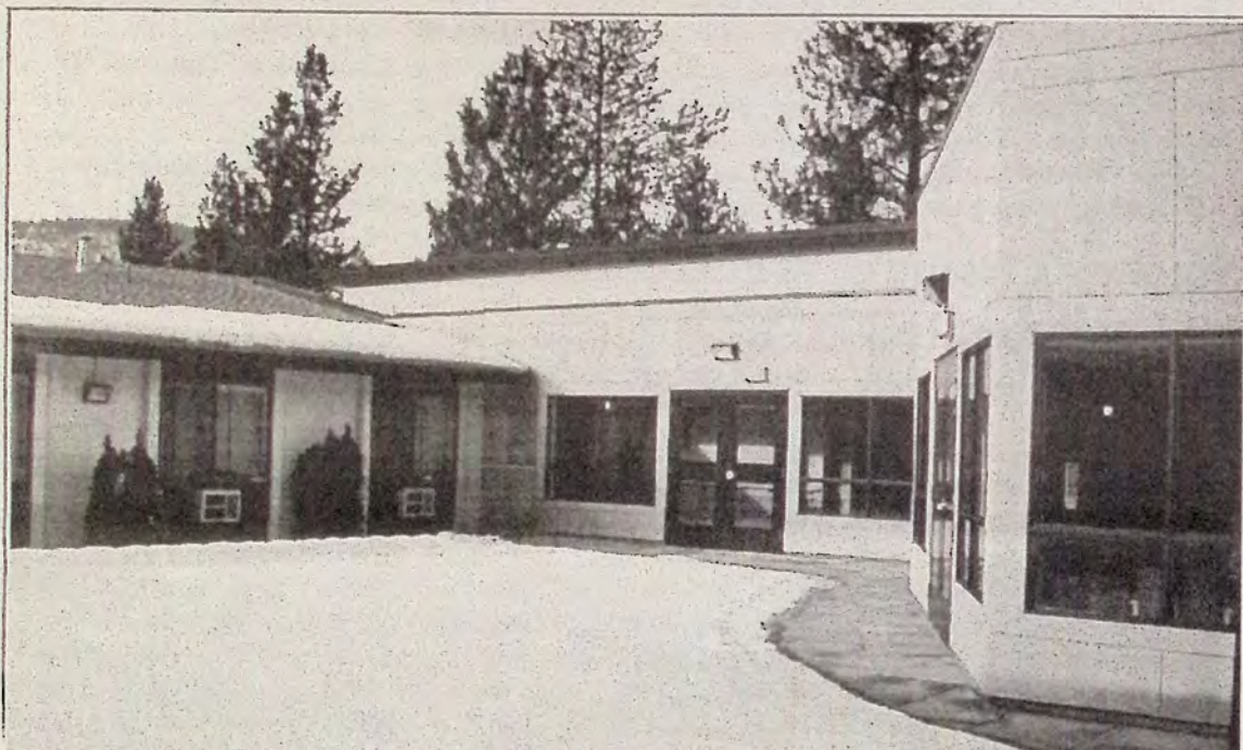
This is the inner courtyard formed by the new wing at Ridgewood Lodge.
