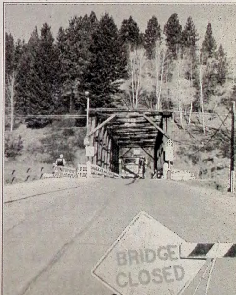
The wooden bridge was closed last Wednesday morning while the Town crew hosed away the last gravel of winter.
