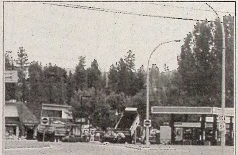
The paving project on Bridge Street kept everyone busy trying to find where the detours were, but Princeton Esso joined in the paving project on Friday morning to improve the appearance of their self-serve drive-through.
