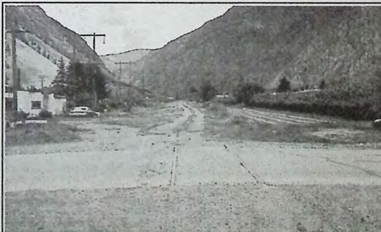
BC Gas proposed right of way follows the old Great Northern Railway route through Keremeos.
