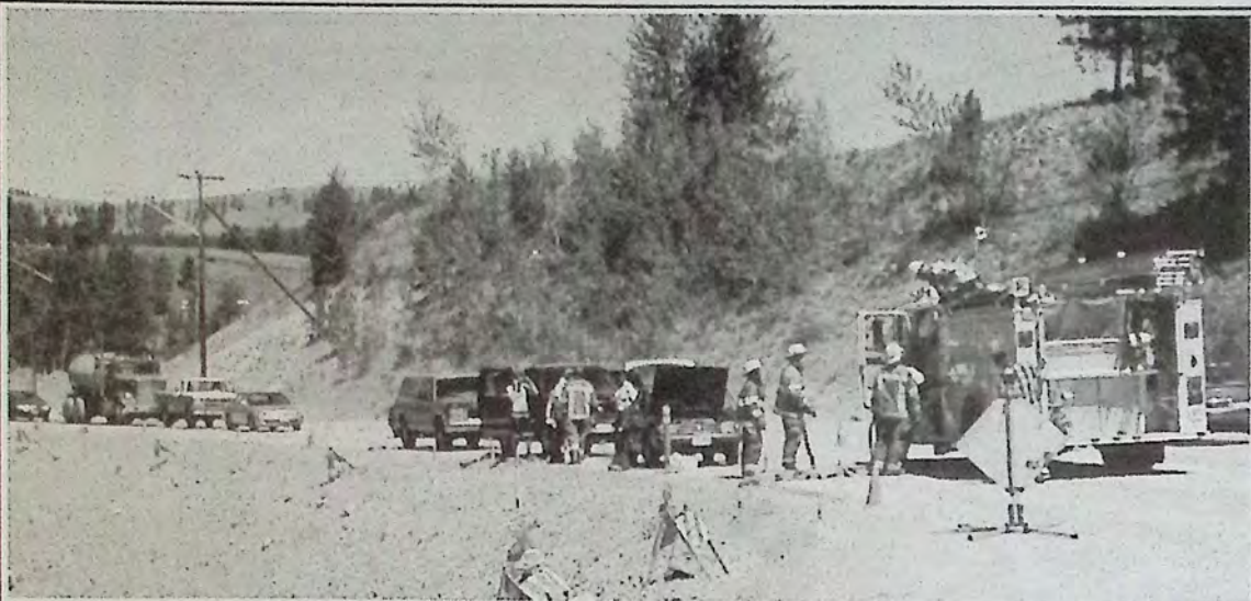
Line-ups to the new bridge during paving last week were extremely hot. The line-up one day was further complicated by a car catching fire and the Fire Department arriving. The heat was nearly unbearable for drivers, and nobody could understand how the flagpersons and paving crew could endure the exposure to the high temperatures for an entire shift.
