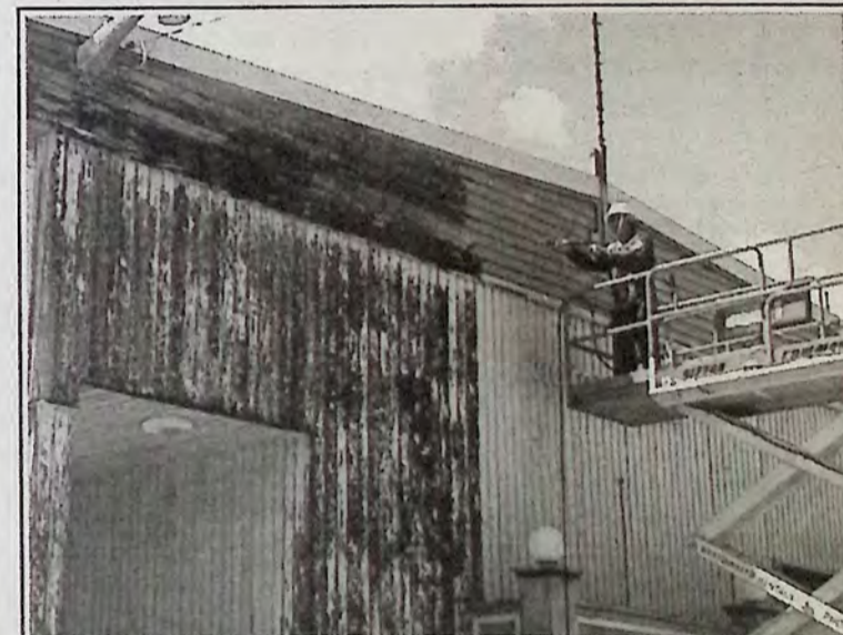
Public Works foreman Bob Stanley pressure washes Victory Hall in preparation for a new coat of paint for the old building.
