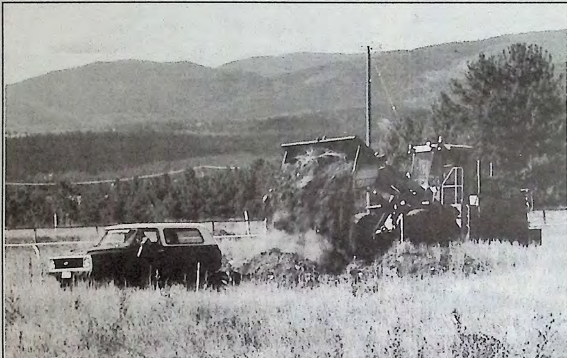
Tuff Truck track construction began Saturday.
