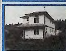
Back to back 2-storey duplex located right downtown. Rear unit rented at $550 per month. 5 appliances with each unit. 7 years old with a nice floor plan. Live in one side and have the other side pay your mortgage. Call HEATHER JOHNSON to view. $109,000 MLS
