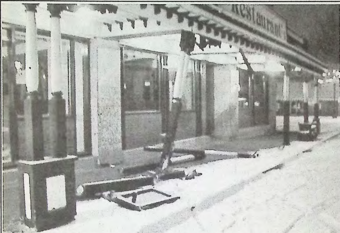
The facade of Princeton Hotel suffered substantial damage when a vehicle drove through the posts supporting the canopy. Note the tire tracks on the sidewalk.
