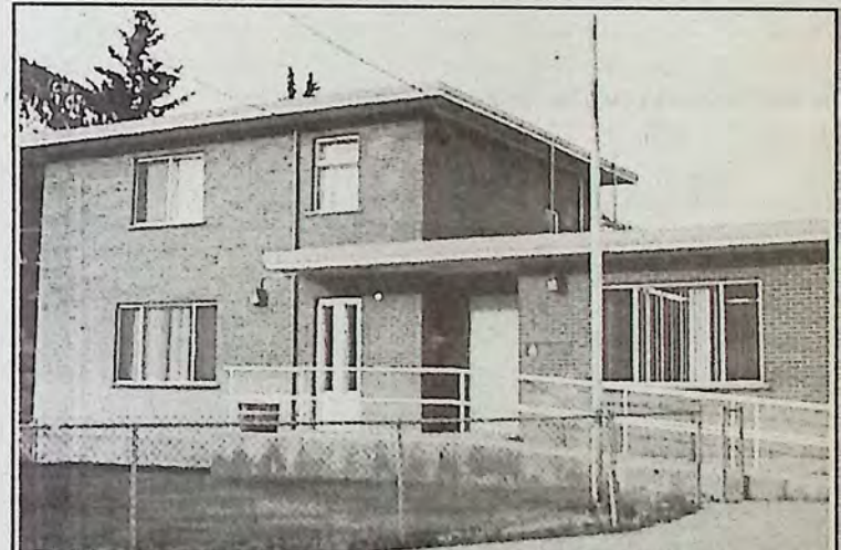
A new RCMP station will be built in Keremeos next year. Construction is slated to begin in February 2004. Planning ahead, Village Council has asked that the new building be designed so a fire hall can be added on. There is adequate land to do this, and Council is looking at the time when the present fire hall must be replaced. Council's wish is being considered. The new building is in the design stage now.
