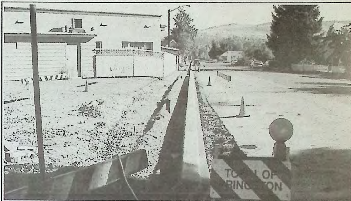
The much-needed new sidewalk on Halliford Avenue is in the works.
