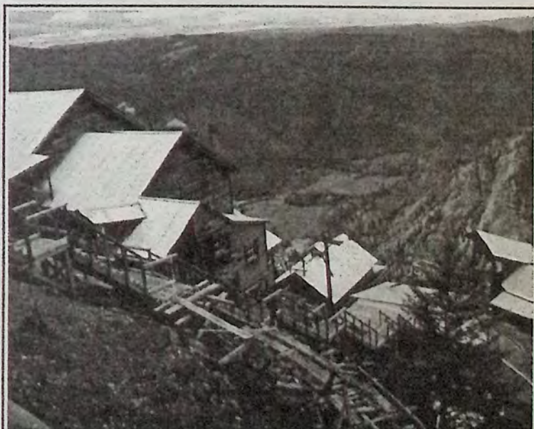
The wooden stairway contains landings and benches so visitors can take their time and enjoy the scenery.
