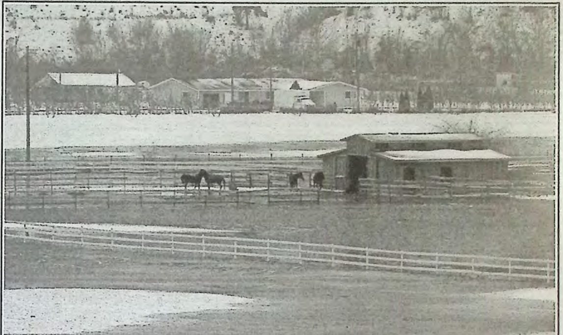
This is the view of one of the flooded fields on River Road in Keremeos. A work party has been organized to help clear away ice and debris at Don & Anna's Greenhouses, which was hit hard on January 19th. Volunteers wishing to help can contact Judy Egli at (250) 499-5681. The plan is to have 12 volunteers a day on site until the job is done. Volunteers are asked to pre-register. Photo: Bryan Smith, www.keremeos.net
