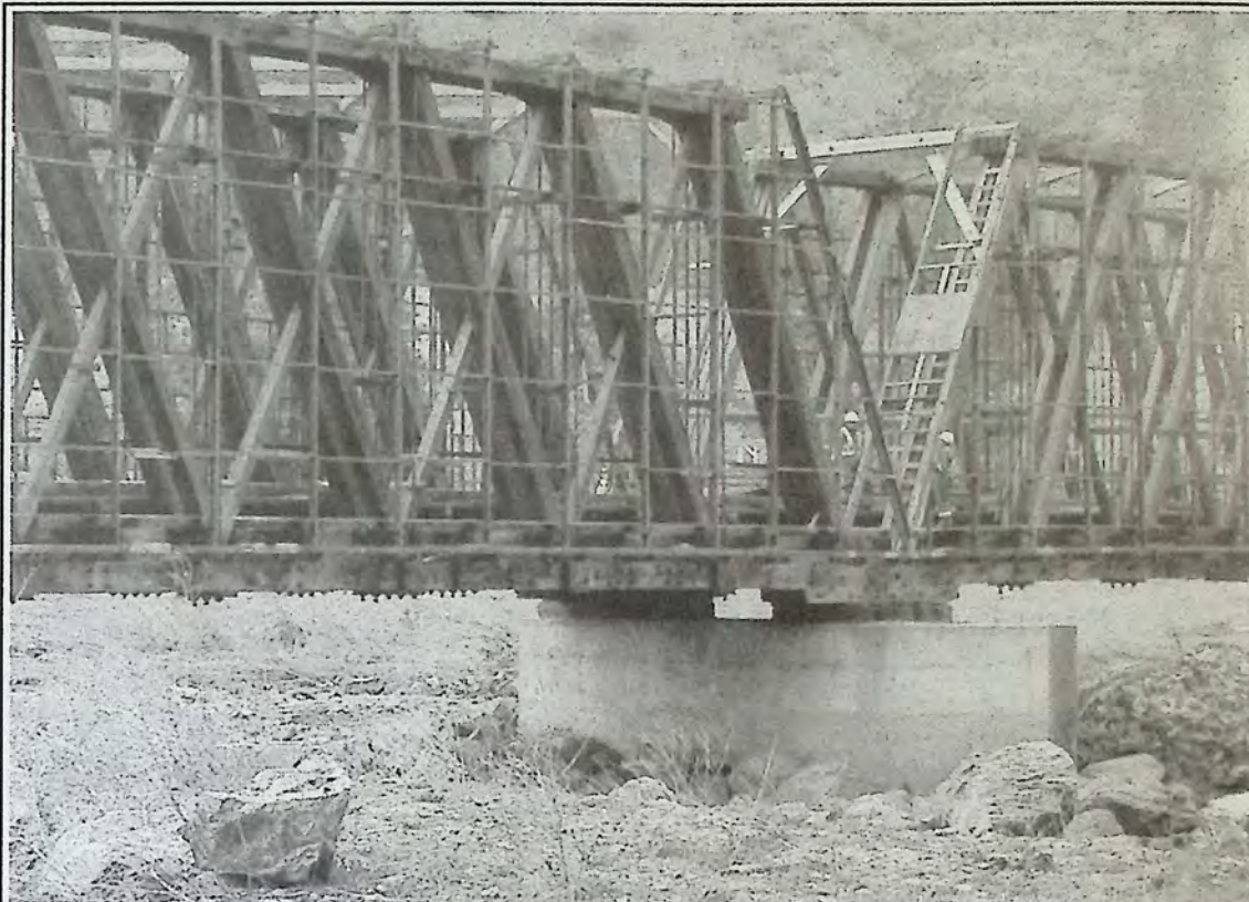
The historic red bridge at Keremeos looks nothing like we are accustomed to without its cladding.
