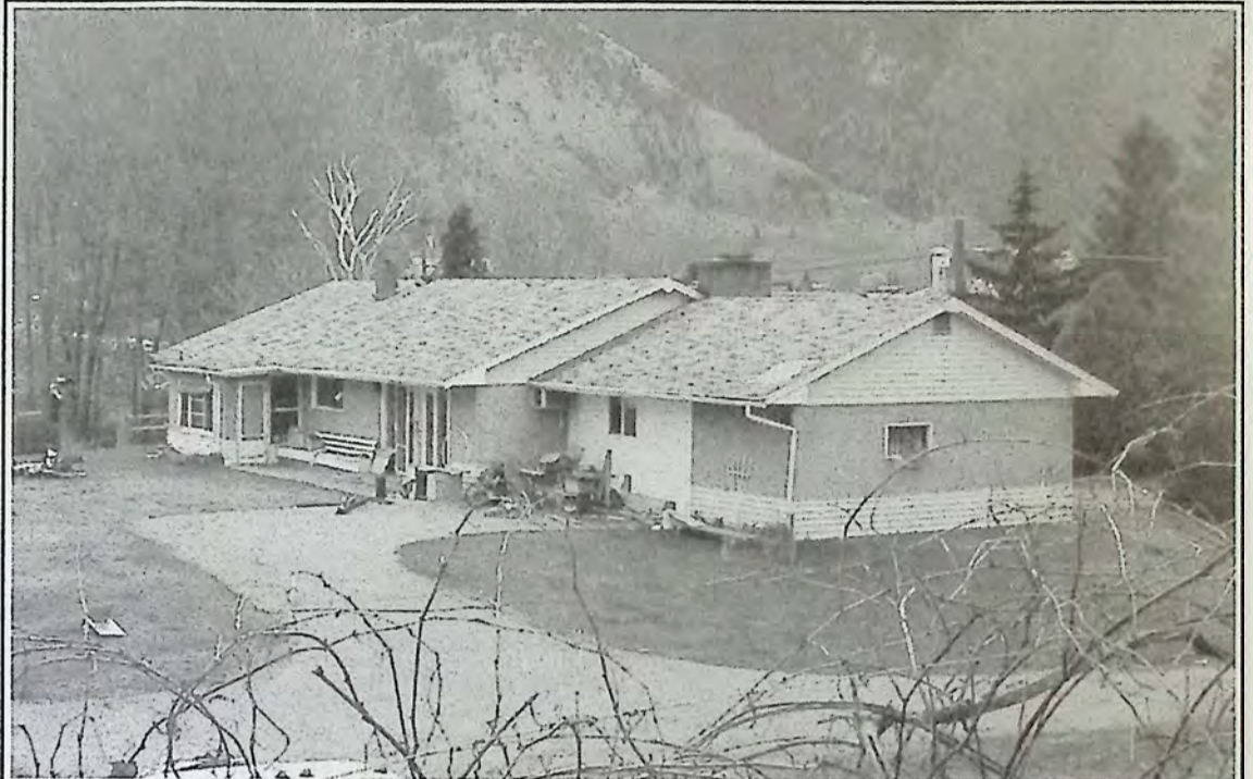
This was the home that suffered serious structural damage resulting from a fire on April 10th.
