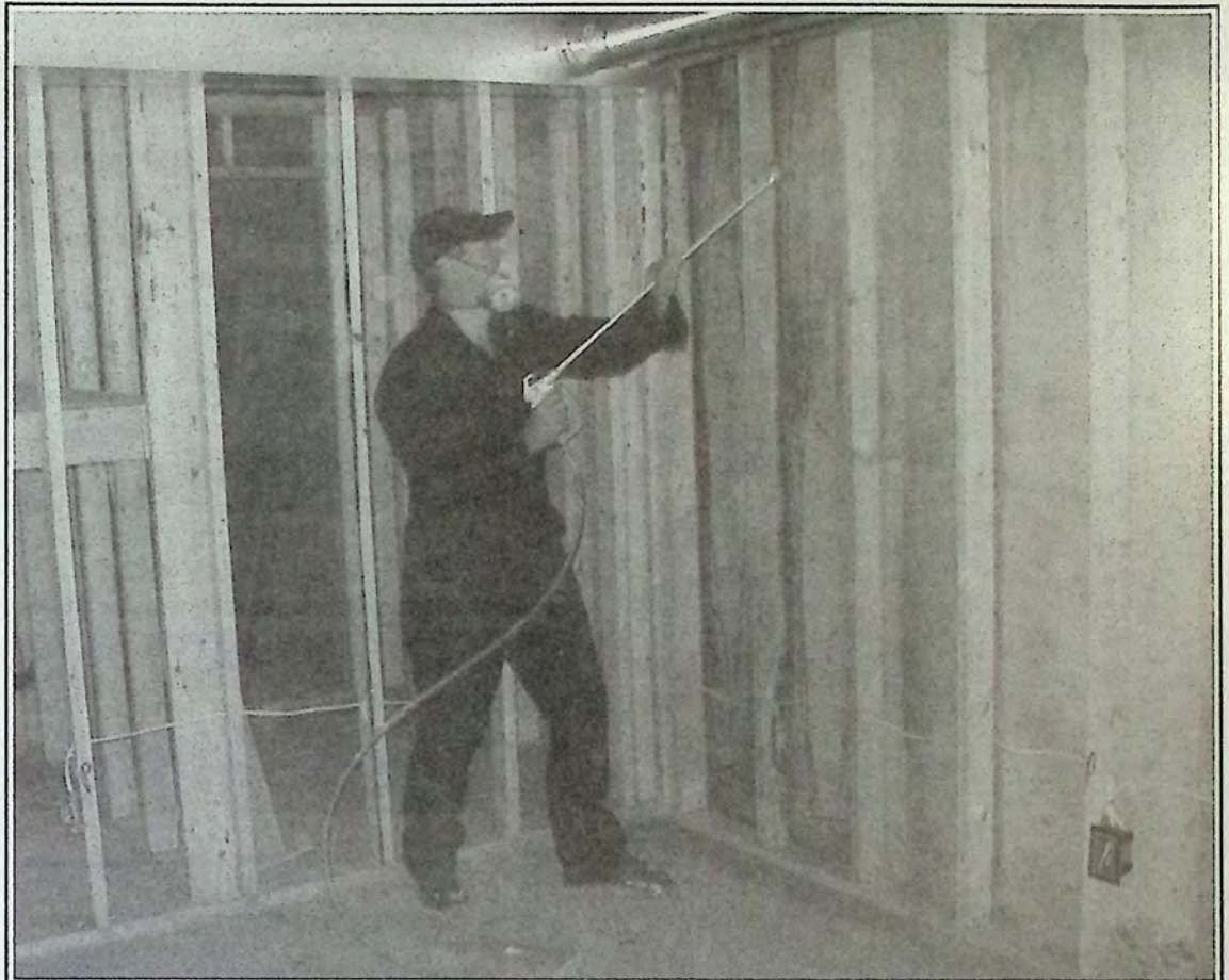
No-Burn Canada President Mark Harrison applies his No-Burn product to the basement of a new home on Coalmont Road. The demonstration introduced the product to British Columbia.
