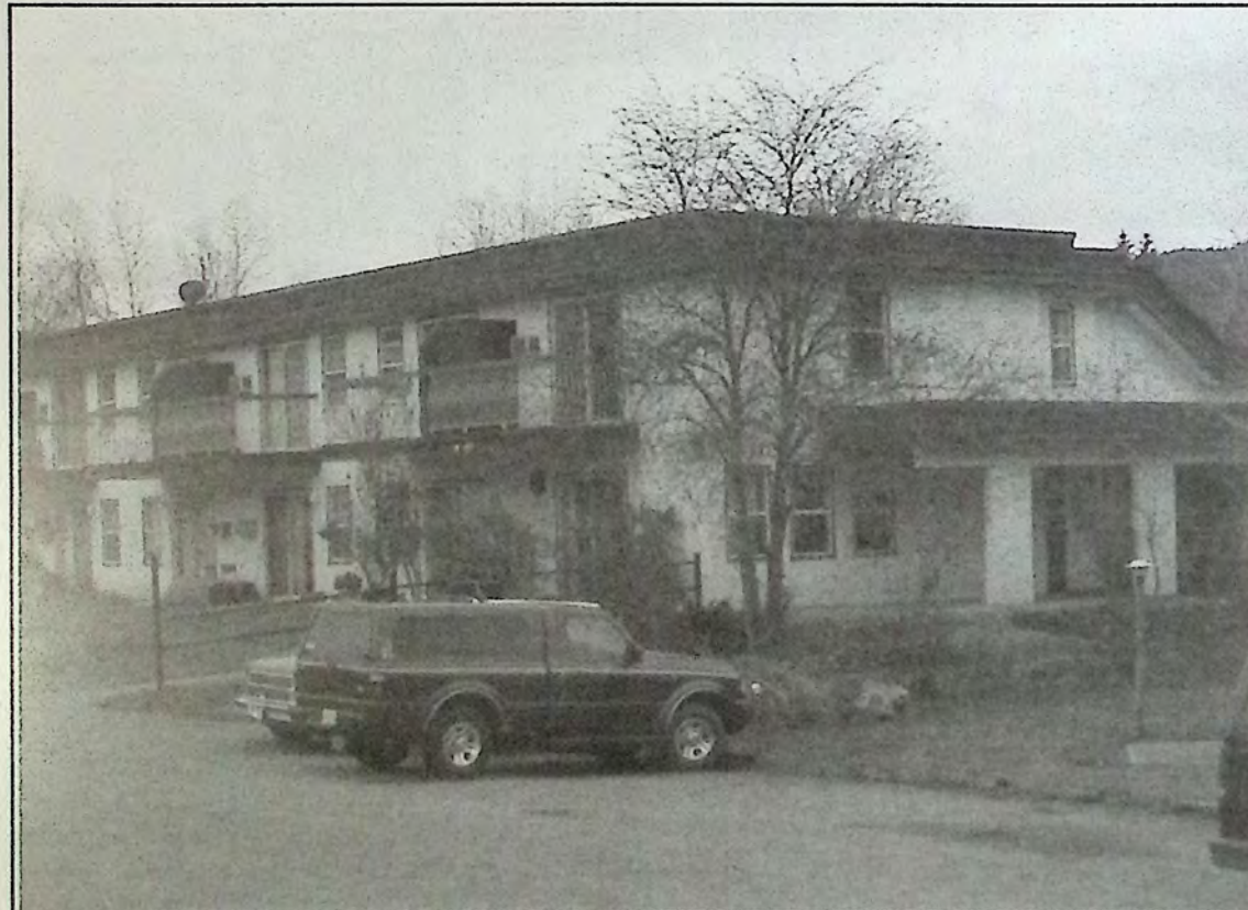
Silvercrest Housing Development is located in downtown Princeton, overlooking the Tulameen River.
