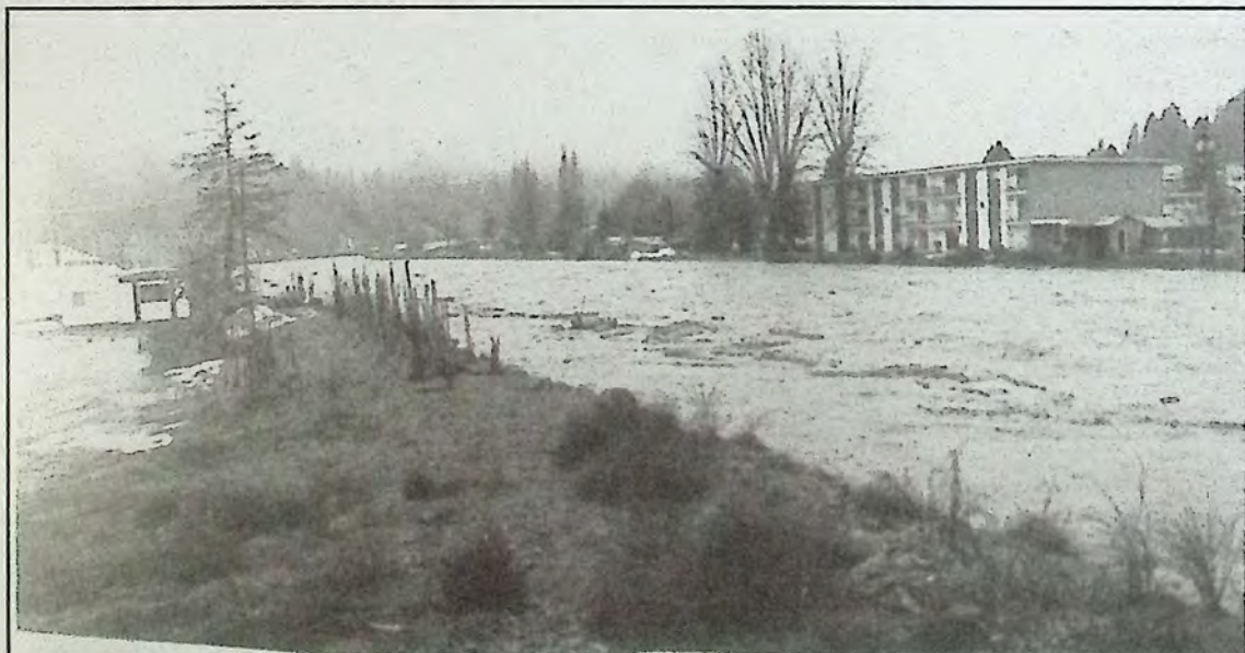
The Tulameen River reaches the top of its dyke.
