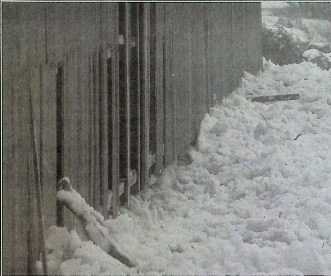
The historic red bridge near Keremeos took a beating during the ice jam of January 19, 2005. Although some boards were already missing before this photo was taken, the ice build up damaged many more. Photo: Bryan Smith, www.keremeos.net.
