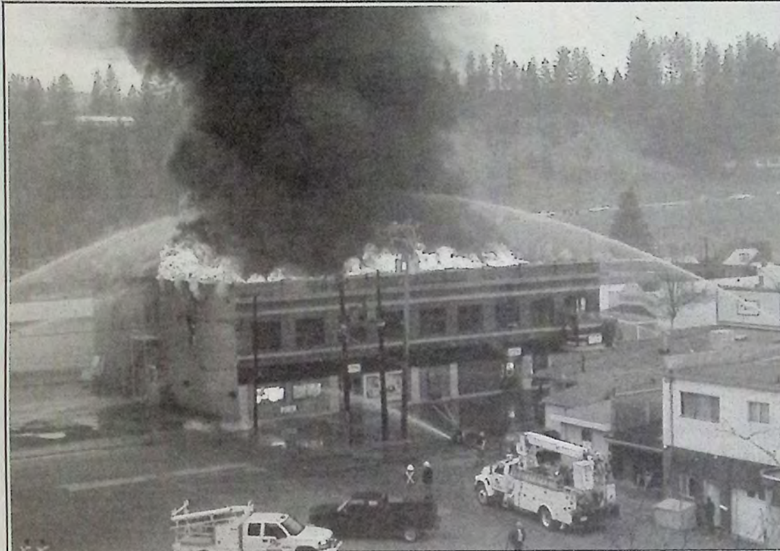
Princeton lost a landmark early Saturday morning when the Princeton Hotel was destroyed by fire. The brick building, built in 1910, was the oldest building in downtown Princeton.
