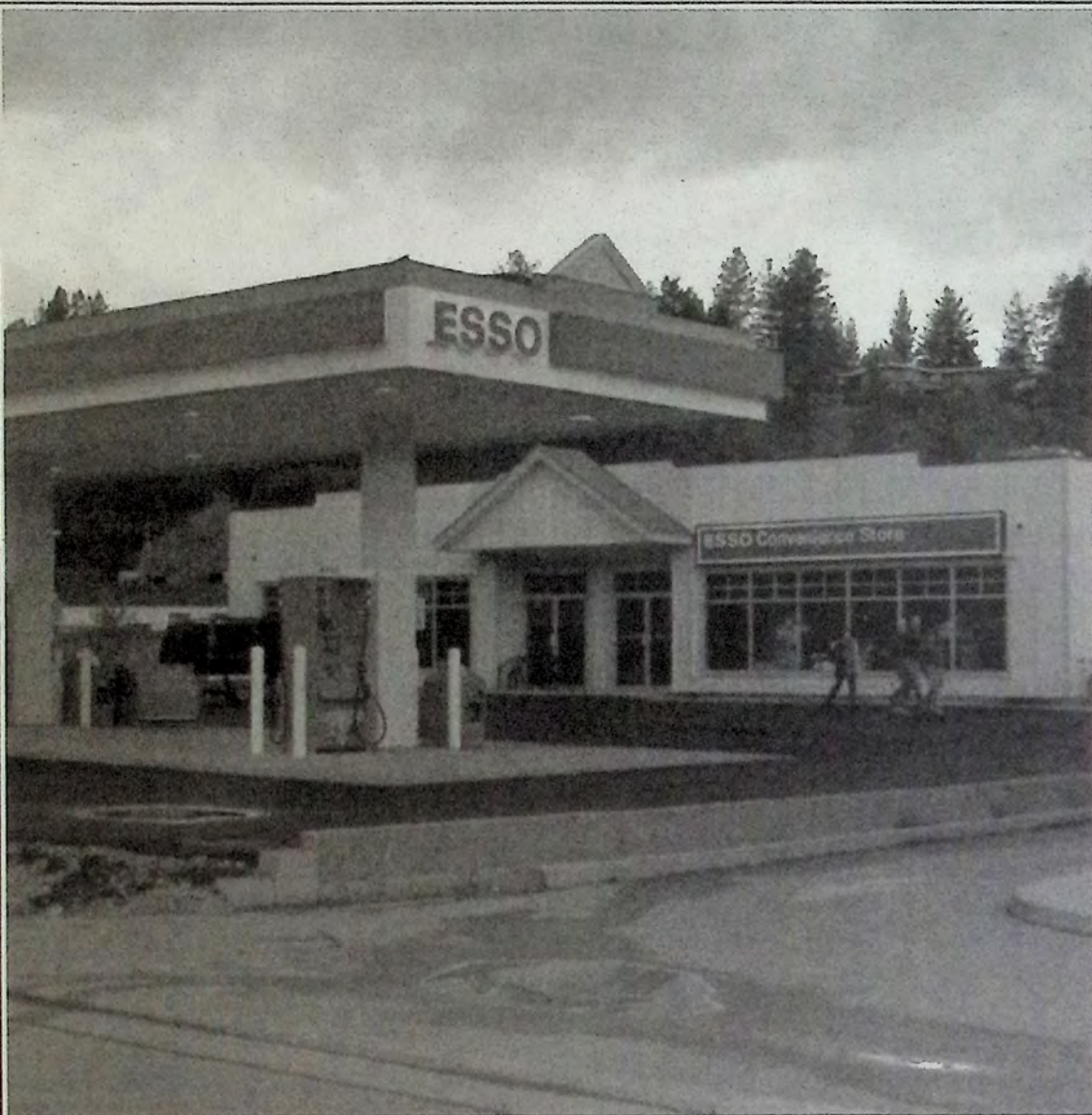
The piece of commercial property on Highway 3 between Dairy Queen and the Best Western took a long time to sell. Construction of the new Esso Service Station/Convenience Store at that location took a long time to complete, but it finally opened for business last Wednesday. We welcome the new Esso to the local business community and are pleased to announce they will also have the Similkameen News Leader available at their in-store news stand. Watch for an official Grand Opening to take place soon.*
