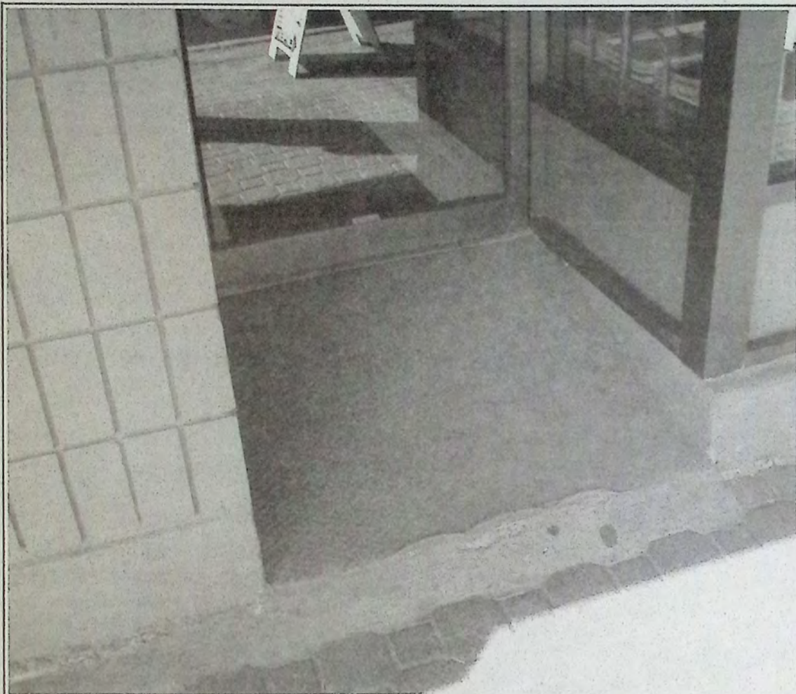
We used to be pretty proud of the fact that our downtown office had a ramp leading to the front door - that is, until we discovered it is far too steep a grade to be inviting for some people to use. *
