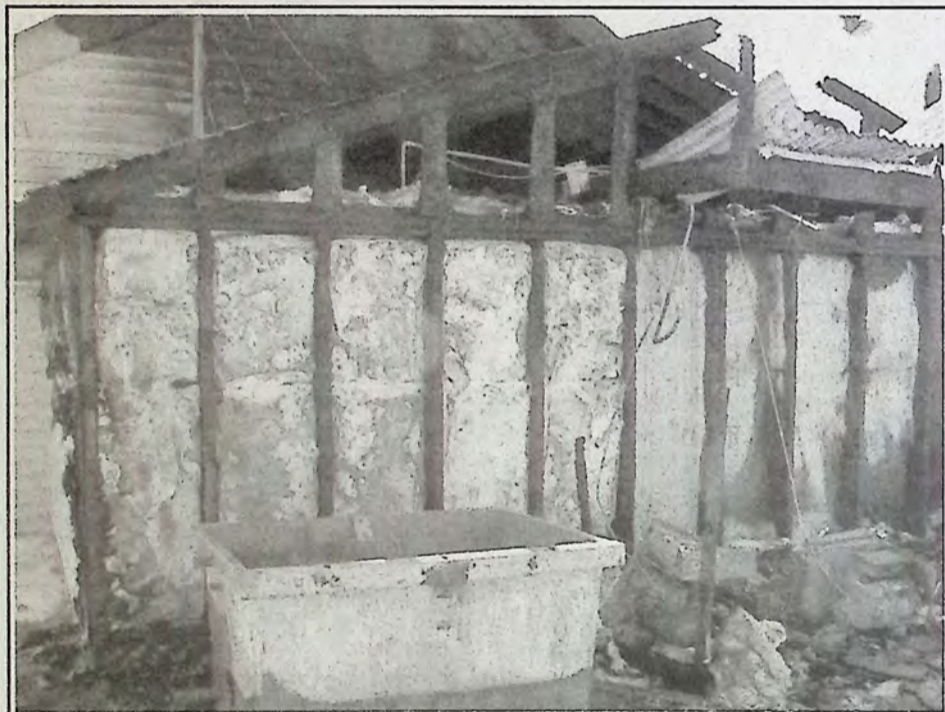
A closer view of the back of the restaurant building.*
