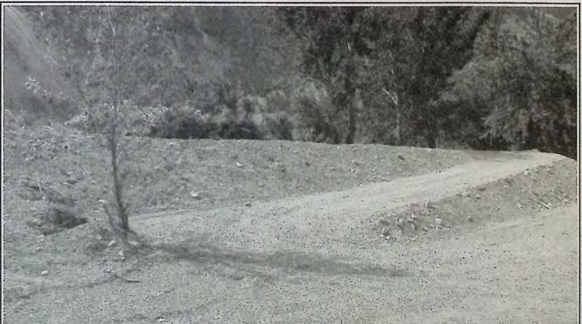
This wheelchair ramp provides access to the Keremeos Promenade, a loop walking path that follows a portion of the Similkameen River dyke and KVR right-of-way, created by the Village of Keremeos and the Similkameen Trails Society. The Promenade was officially opened in a ceremony on July 1st. *
