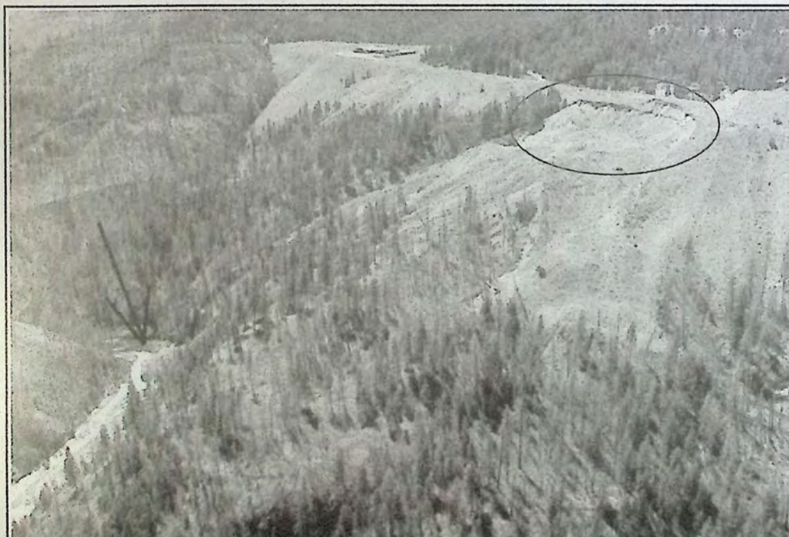
The circle shows the top of the slope of tailings that were part of the landslide into the Similkameen River August 1st. Arrow points to the location where the river was blocked. Okanogan County Sheriff's Department Photo
