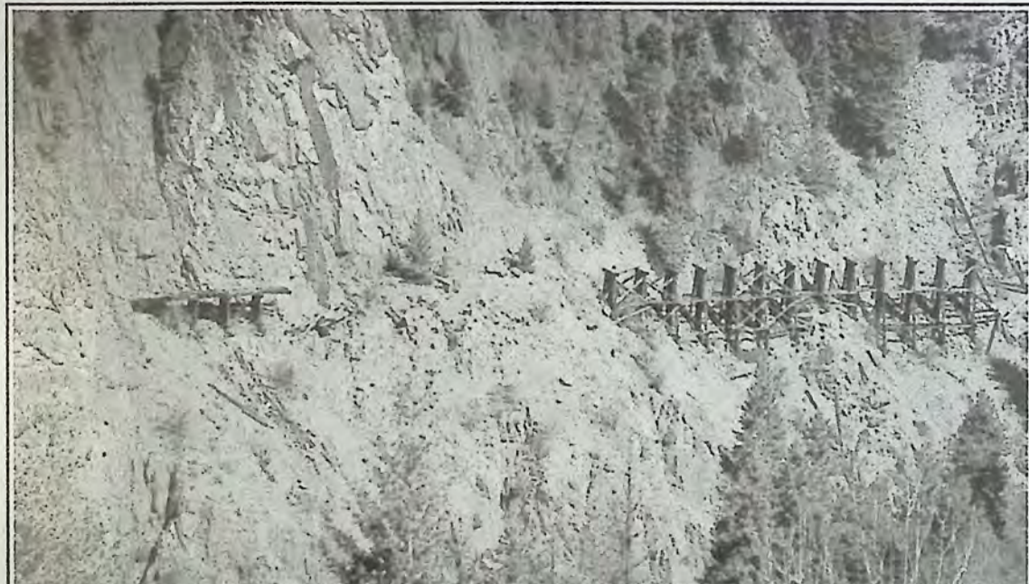
The incredible engineering feat of the Copper Mountain Railway can still be seen in places along the Similkameen River. The transportation route was used for many years before it was abandoned.
