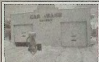
285 Bridge Street Business located in high traffic area. MLS 43213 $219,900
