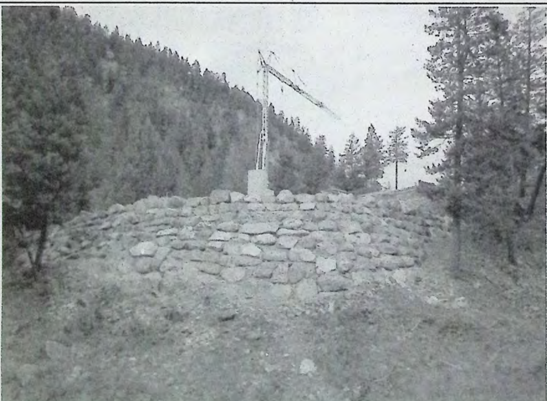
Construction continues as RockRidge Canyon grows and expands.*
