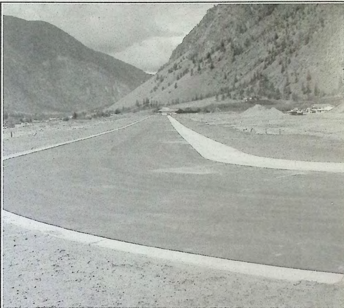
The view from K-View Estates looking West towards Princeton. *
