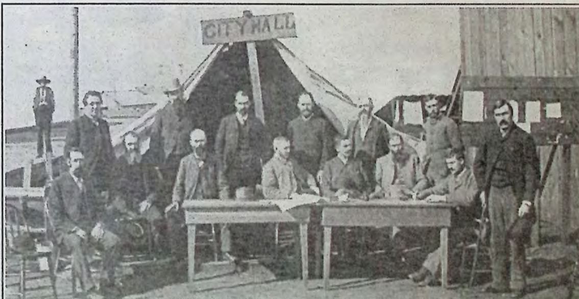
Vancouver City Hall following the fire. - photo submitted
