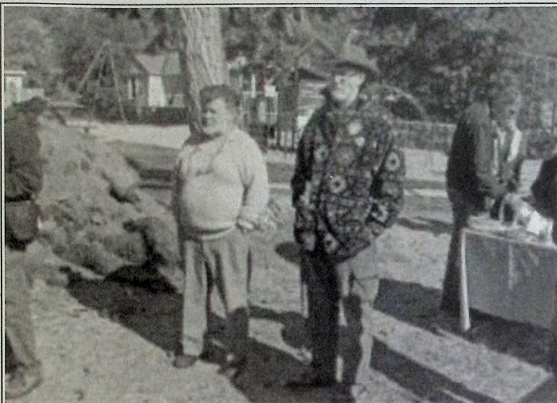
Woodlie Park Project Manager Elef Christensen, left, and BC Southern Interior MP Alex Atamanenko attend the sod turning ceremony October 10th. - photo submitted
