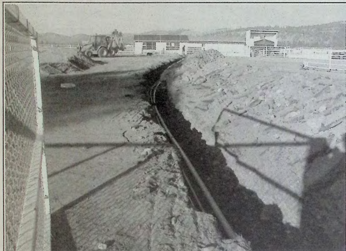
What looks like a bad case of gophers is actually work being done at Sunflower Downs to move water lines and power service underground. This is the view across the race track and into the rodeo arena. *
