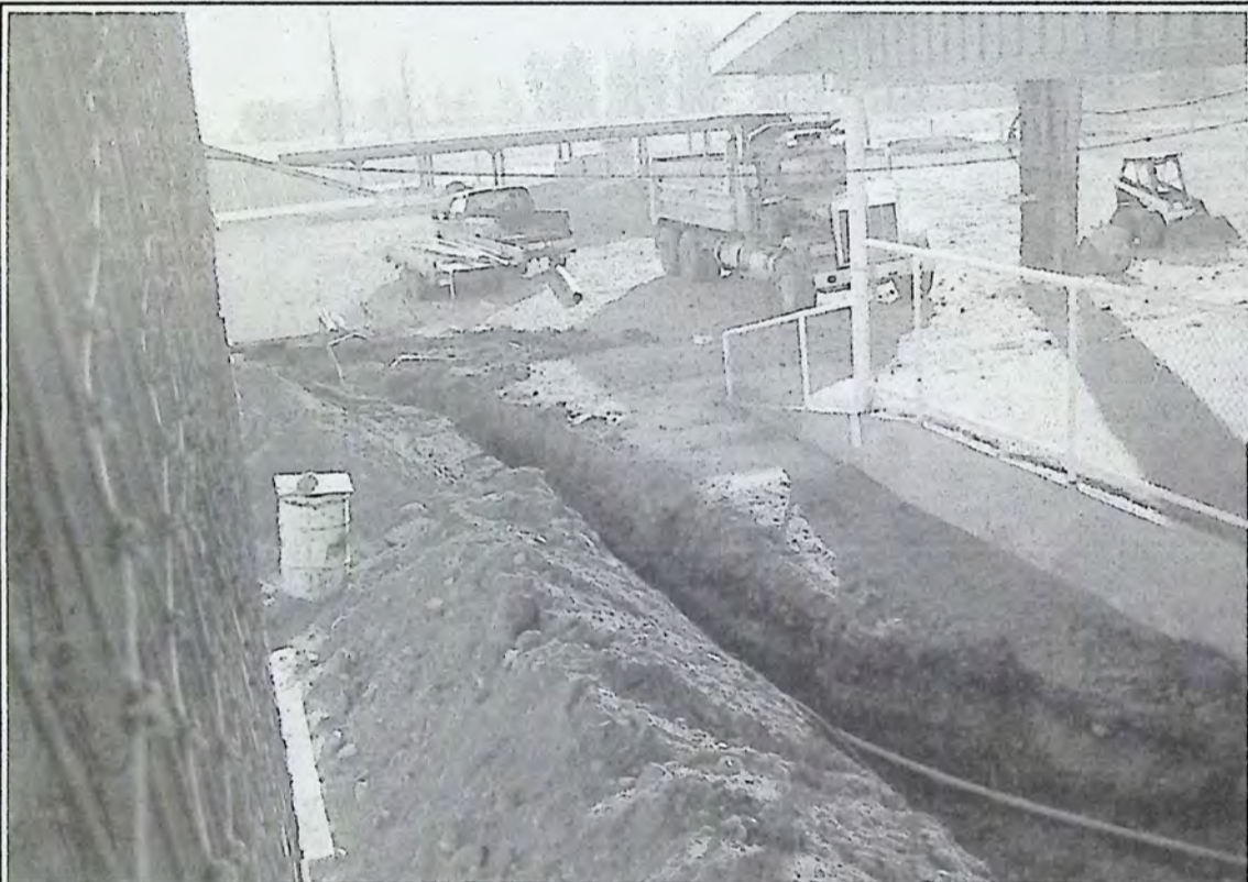
The view between the grandstand building and concession. *
