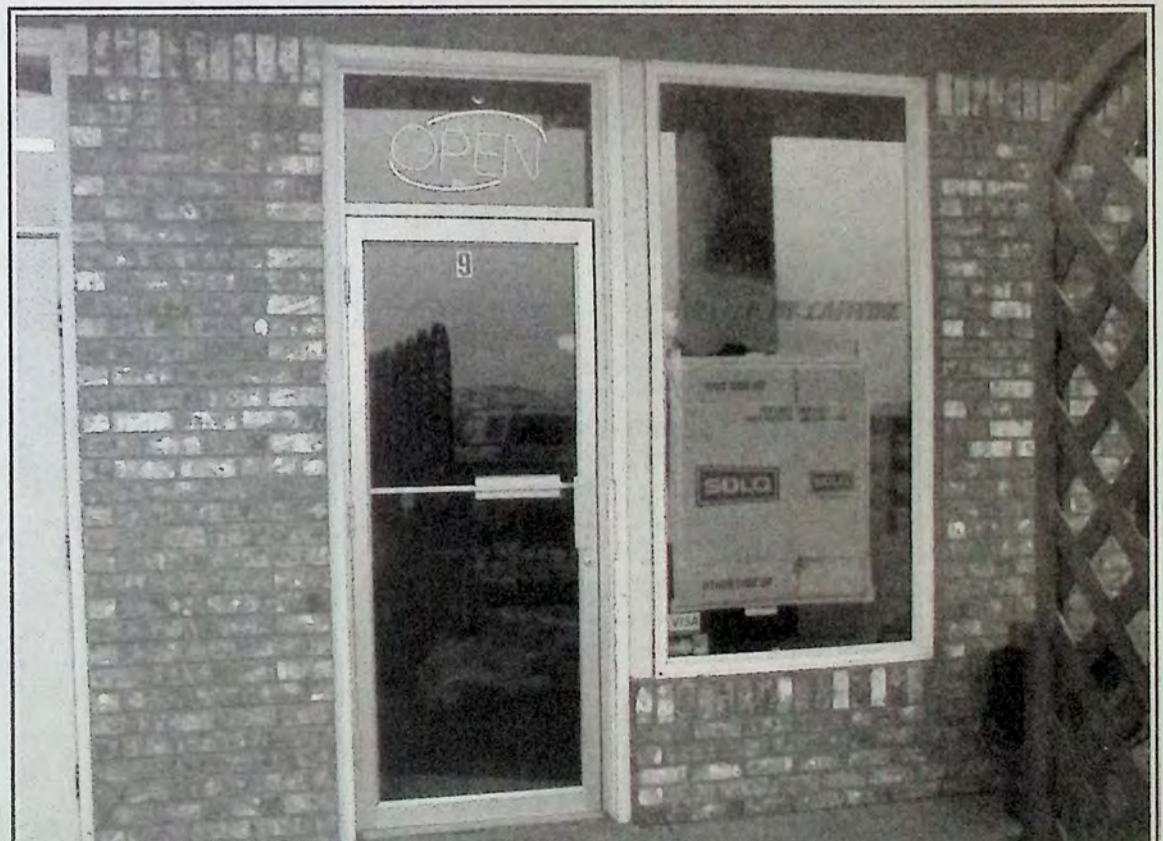
The front window at Cowboy Coffee was smashed last February 3rd along with many other windows in Princeton Plaza and a couple of businesses downtown. *
