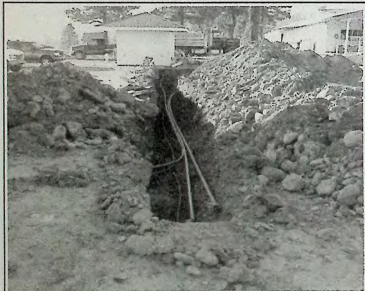
This trench ran in front of the Fall Fair buildings.*
