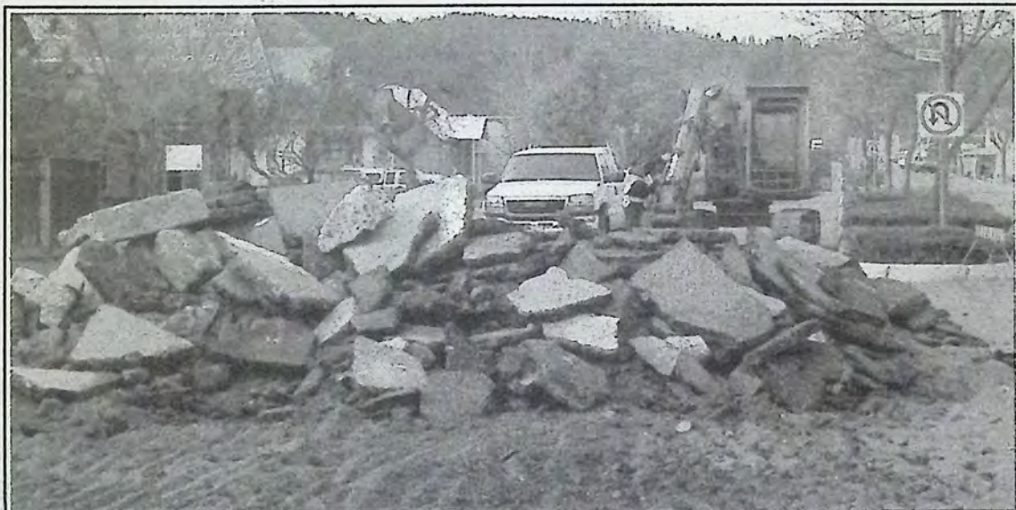
Work resumed last week on the Town Square Project. *
