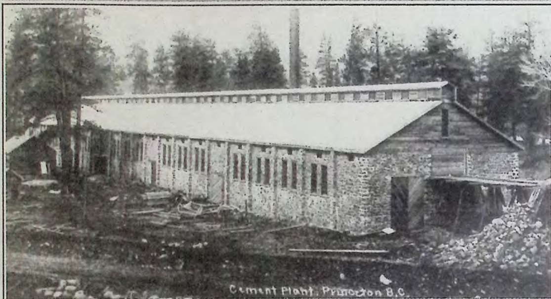
The Princeton Cement Plant while under construction. Photo: Princeton Museum
