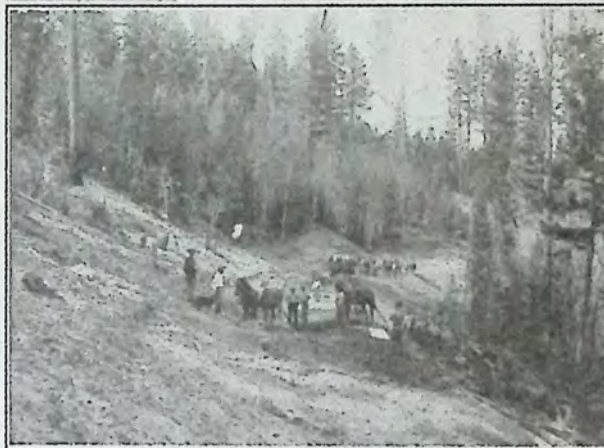
Hope Road Construction 1914
