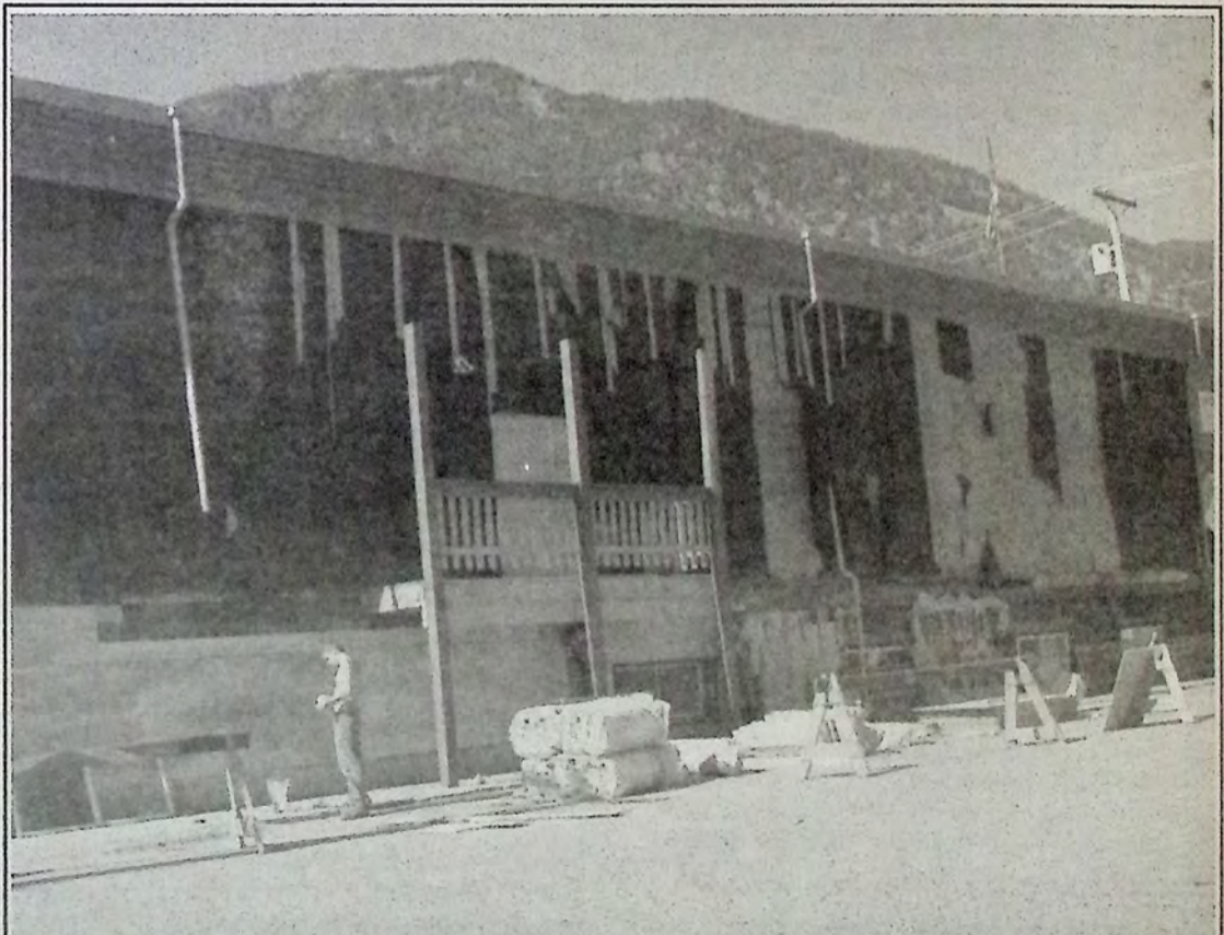
Another look at the Victory Hall renovation project. Photo: Brenda Engel
