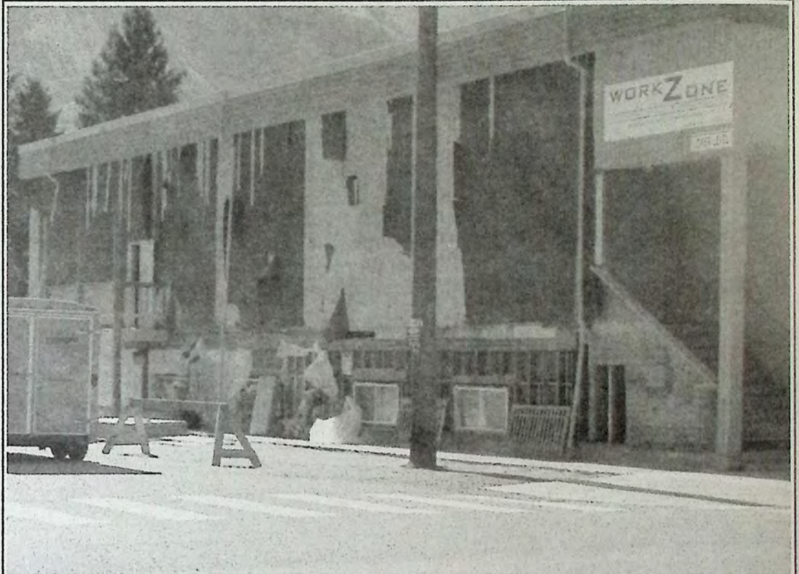
Renovation work on Victory Hall started last week. Photo: Brenda Engel
